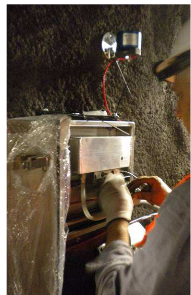
Installation settlement tank
