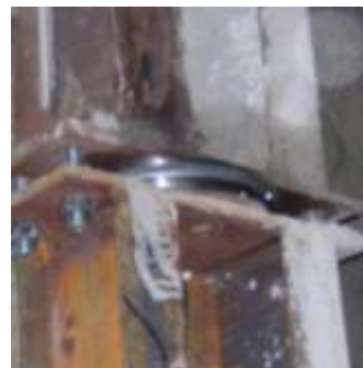
Installation of cell between two elements of a rib
